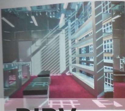
Figure 1. Internal view of ONYX photovoltaic glass-panels curtain at Balcinaga storefront (Minsk). The BIPV laminates include crystalline silicon technology and float glass, one of the products developed and tested within PVSTES project.
