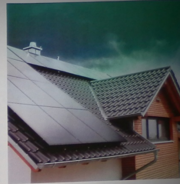
Module clamps and bearing rails anodised in black make for the discreet black appearance of the PV system.
